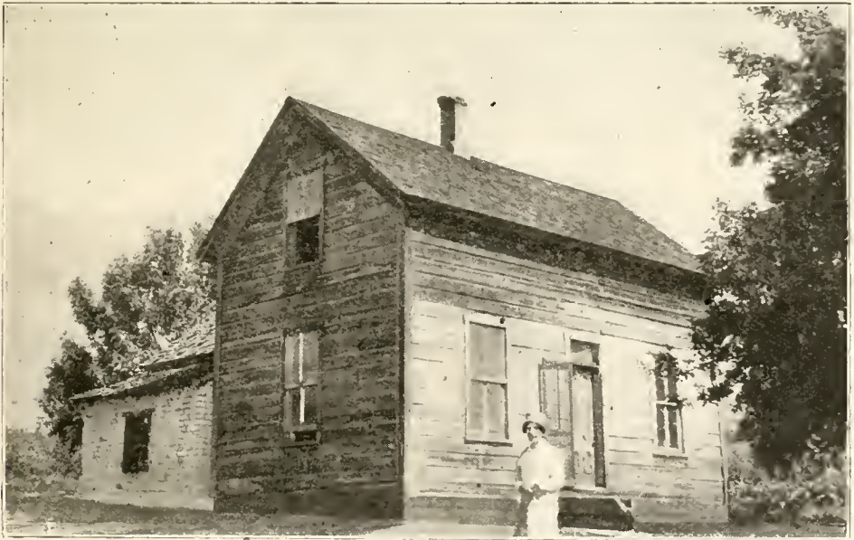
WHAT REMAINS TODAY OF THE OLD JACOB JENSEN HOME IN BRIGHAM CITY. THE INCIDENT OF THIS STORY OCCURRED IN THE ROOM AT THE RIGHT.
